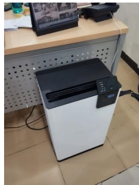
Figure 5 Dehumidifier in Collection Storage Room Source: Researcher Documentation, 2026
