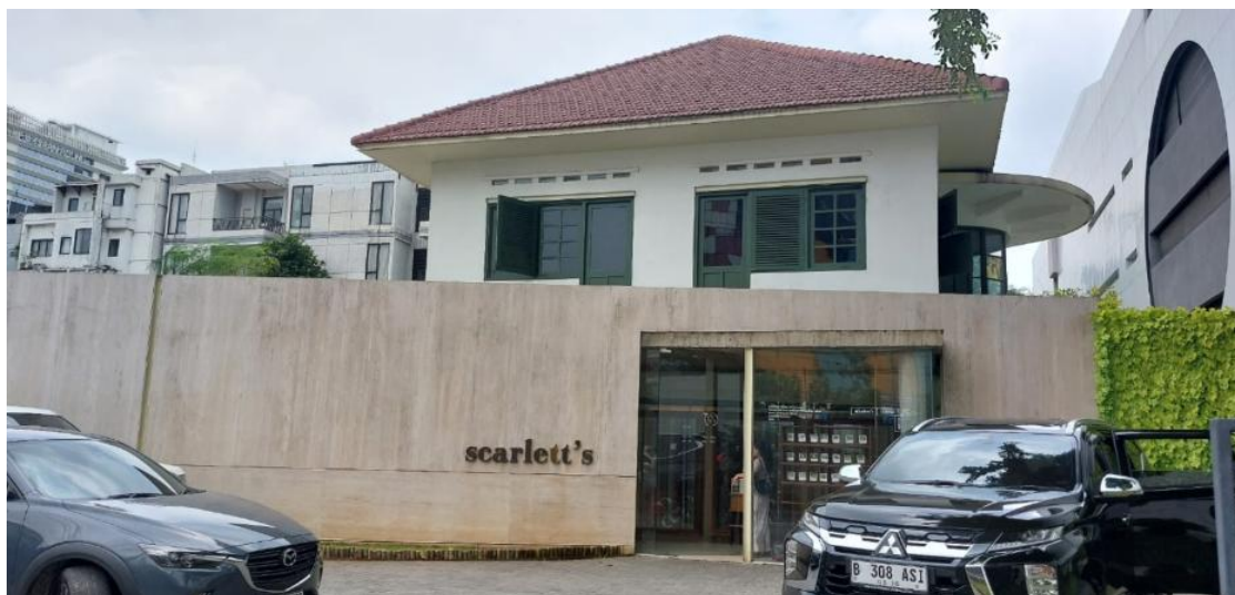
Figure 1. Location of Scarlett's House in Blok M
