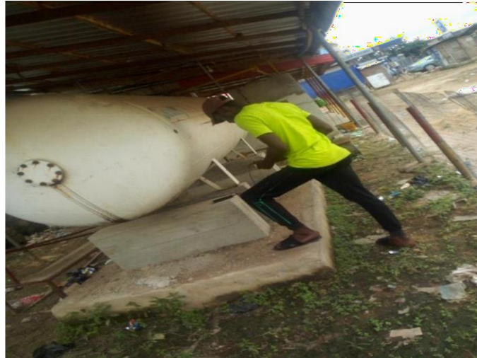
Figure 13. Test carried out at the gas station Source: Snapshot
