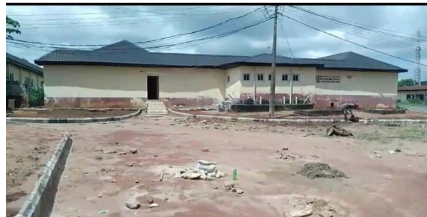
Figure 9: Levelling of driveway area
