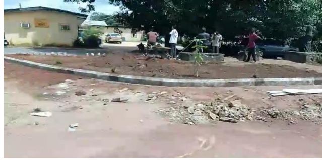
Figure 8: Sand filling and Levelling of Adjacent Area
