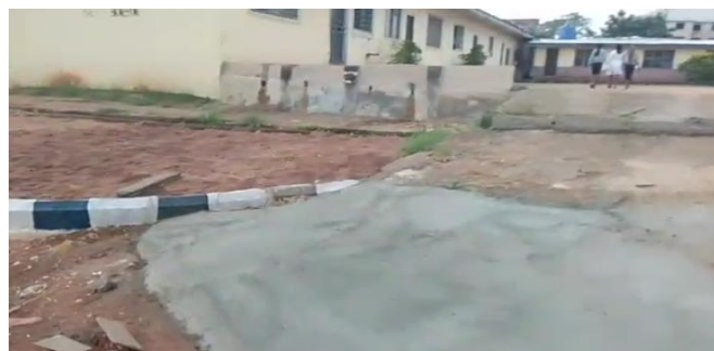
Figure 10: Concrete flooring of AGE/CVE drive way
