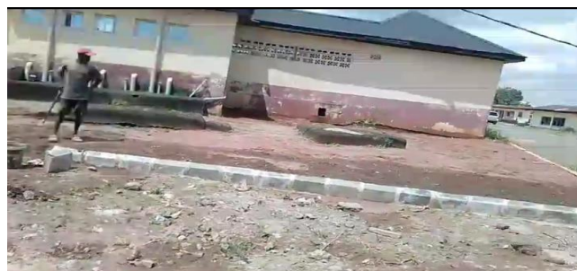
Figure 7: Laying of Kerbs - FENG Area
